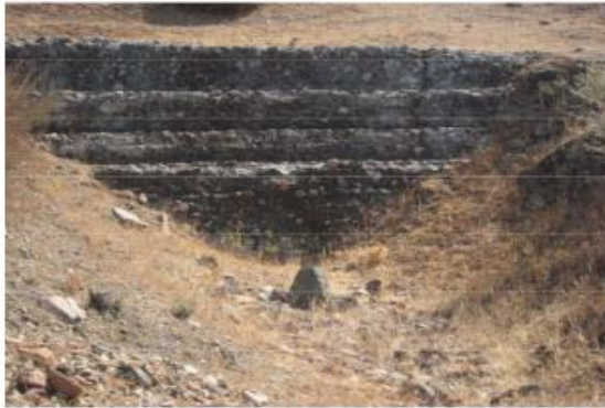
Figure 1: The concrete wall of the Roman cistern at Cerro de La Coja is shaped like a cyclopean and is uneven.
